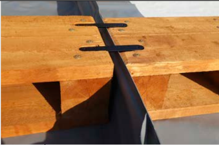
Detail of anchorage of a wooden ramp
