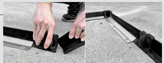
100% impermeability ensured by the silicone sealant used
