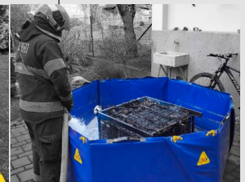
Extinguishing a damaged PV battery storage
