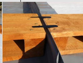
Detail of anchorage of a wooden ramp
