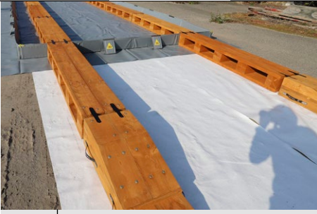
Pool with wooden ramps
